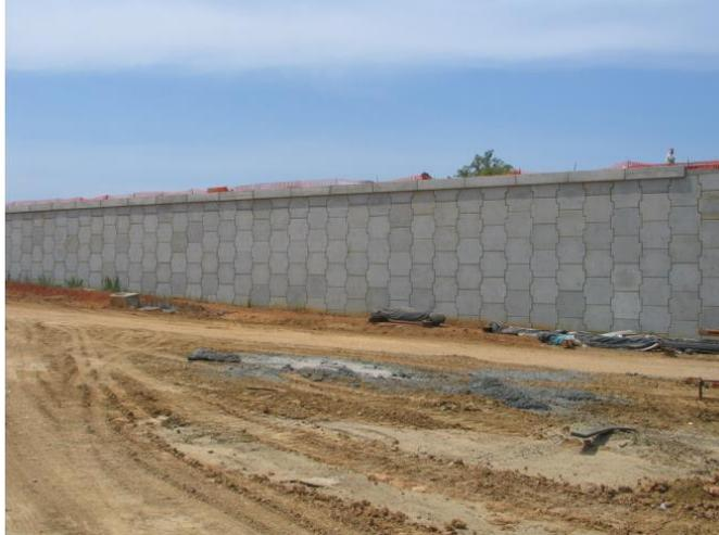
**Figure 1: Example of a MSE Wall**
